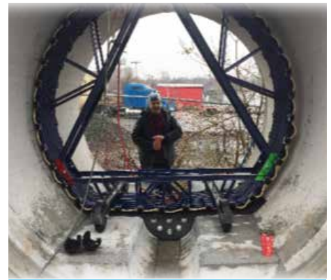
Packer for pipe 96" pipe with cunette
