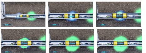
From the cctv/grout truck, the technician controls the equipments used to position, test & seal the joints & lateral connections that fail the air test. The two component low viscosity liquid grout is pumped through the inflated packers and mix in the packer /pipe void where they are forced out through the pipe defects into the surrounding soils to fill voids and form a gel/soil watertight matrix.
