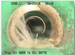
The most common chemical grout used to remotely seal pipe joints, lateral connections and laterals is acrylamide. Having a very low viscosity (1-2 cps), PR 10 acrylamide grout can easily be pumped through 600-800 feet of hose & small defects that allow groundwater infiltration.
